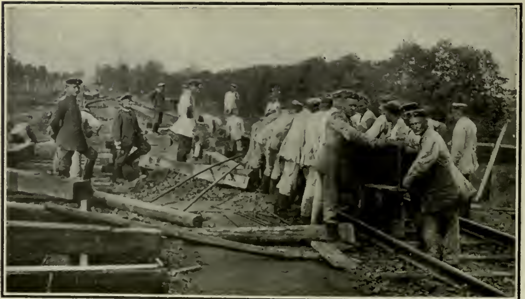
GERMANS REPAIRING THE DAMAGED RAILWAYS IN RUSSIA.
