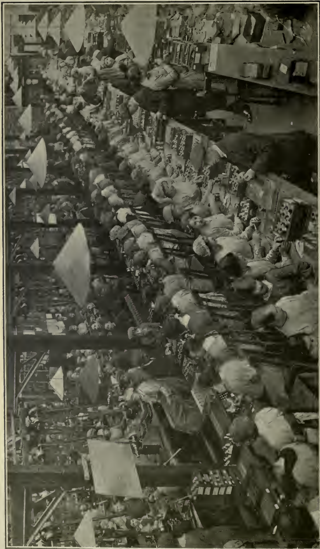
WOMEN AT WORK INSIDE A MUNITION FACTORY ASSEMBLING FUSES.
