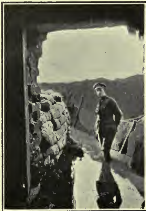
A BRITISH TRENCH.
