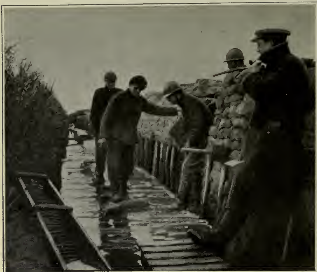
A FLOODED SECTION OF THE BELGIAN LINE, Showing the sandbag breastwork.
