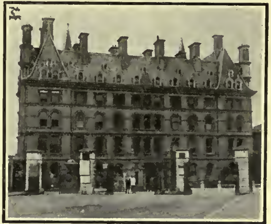
THE STAR & GARTER HOTEL, RICHMOND, WHICH WAS DEMOLISHED.
