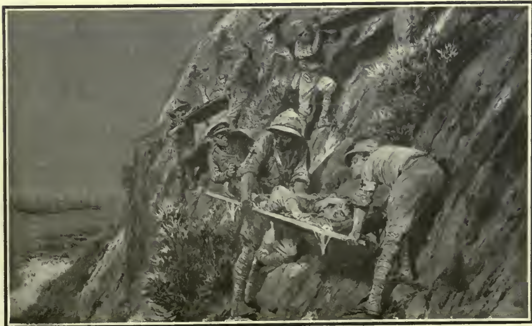
. R.A.M.C. AT WORK: BRINGING WOUNDED DOWN A CLIFF SIDE.
